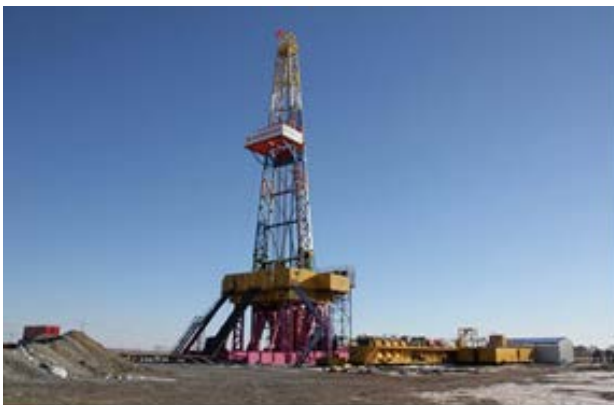
Crust-I, the new Chinese drill rig with 10 km depth capacity
