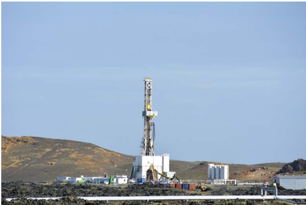
IDDP-2 drill rig near Reykjanes, Iceland. Photo source: Thomas Wiersberg
