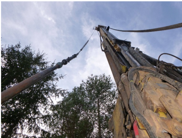
Close-up of the drill rig at S4 Bazina Liba site.
