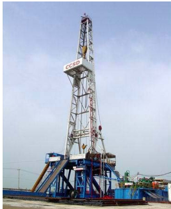
CCSD Drilling in Donghai
