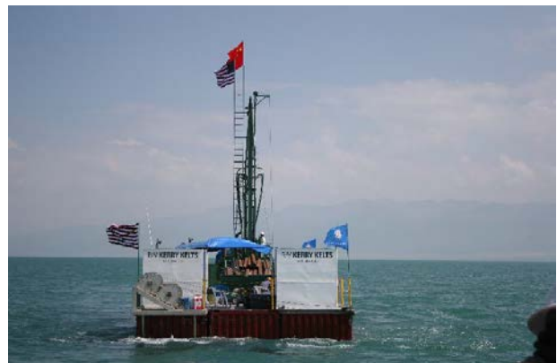
The platform is leaving the base for the drilling site.
