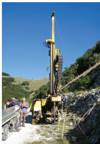
Figure 3. Drilling operations at Poggio le Guaine.
