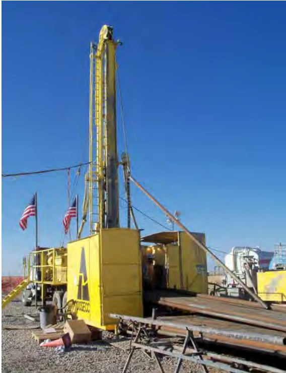
Fig. 4.2.2: Truck-mounted wireline coring rig at Snake River Plain (Project HOTSPOT)
